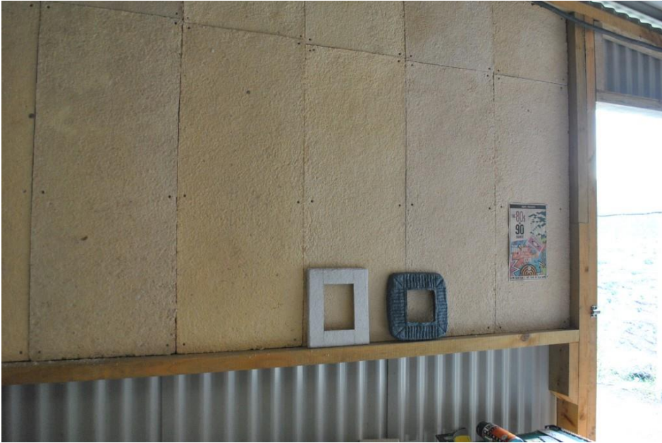
Insulation board trial without borax treatment.
